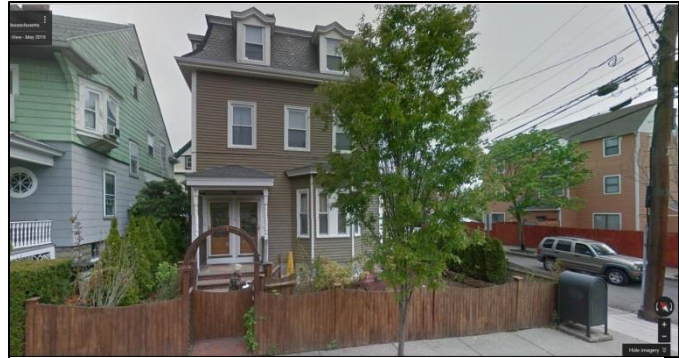
Above: Howe St elevation with old fence.
